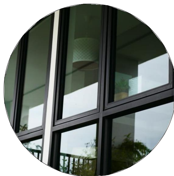
6 TINTED GLASS FOR STOREFRONTS, WINDOWS, BALCONY DOORS VIRACON OPTIGRAY OR EQUIVALENT APPROVED BY ARCHITECT
